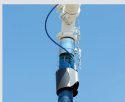
Shut Off valve in pipeline
