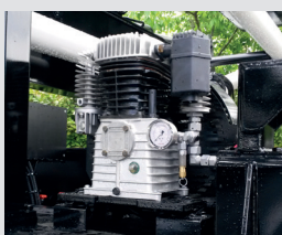
Air compressor for pipeline cleaning
